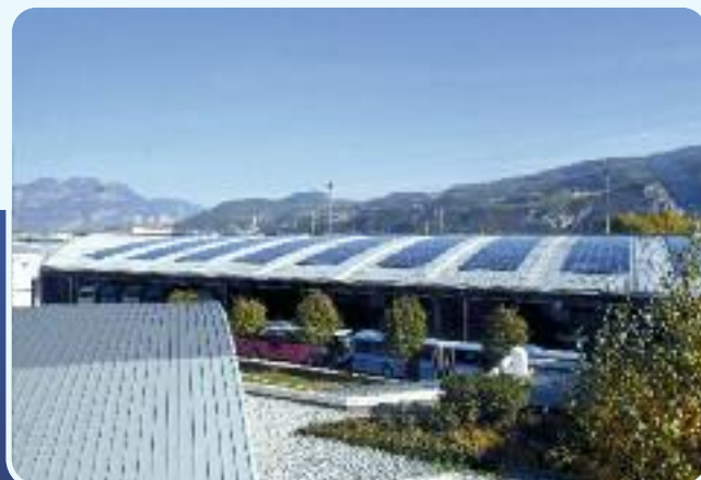
Photovoltaic system for Trentino Trasporti totalling 1,6 MW
