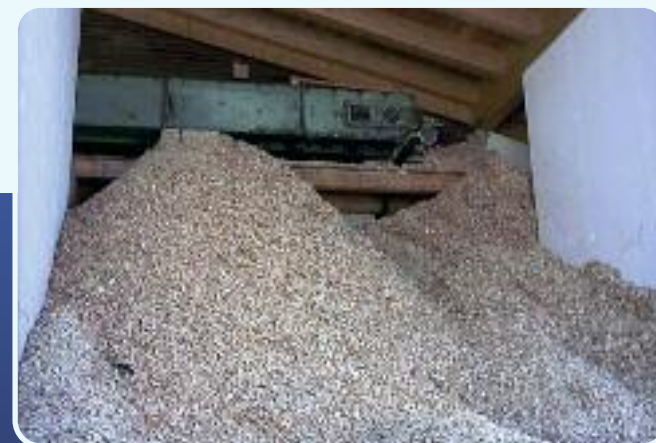
Biomass cogeneration plant of Asiago
